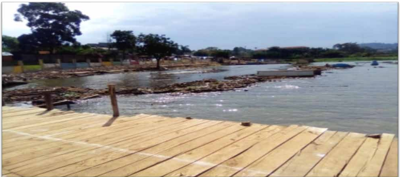
The former Mulungu Market after undergoing “controlled demolition”
