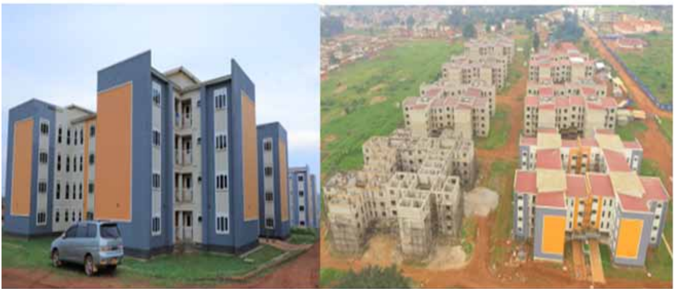
Part of the accommodation apartments undergoing construction
