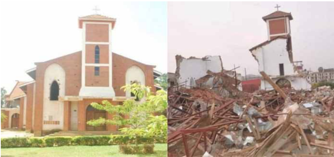
St Peter’s Church Ndeeba, before and after demolition
