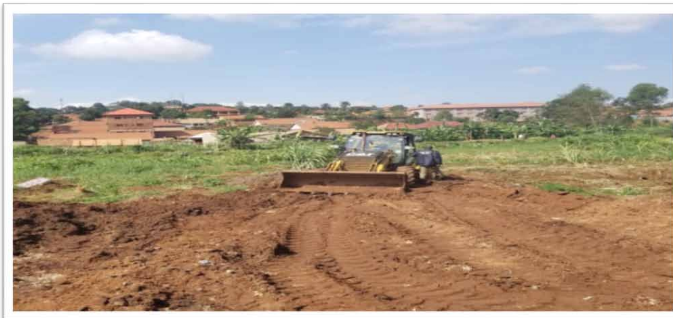
An excavator levelling soil dumped in Kalidubi Wetland System in Makindye.
